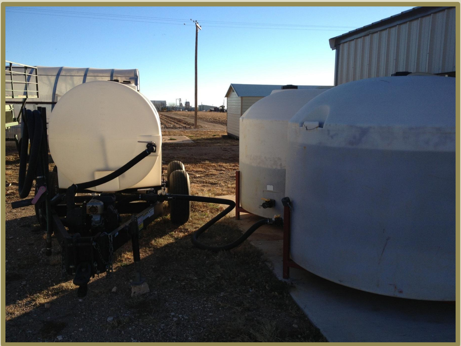
Transfer Tank- A 5.5hp engine pumps waste water from holding tanks to transfer tank where waste water is neutralized prior to disposal.
