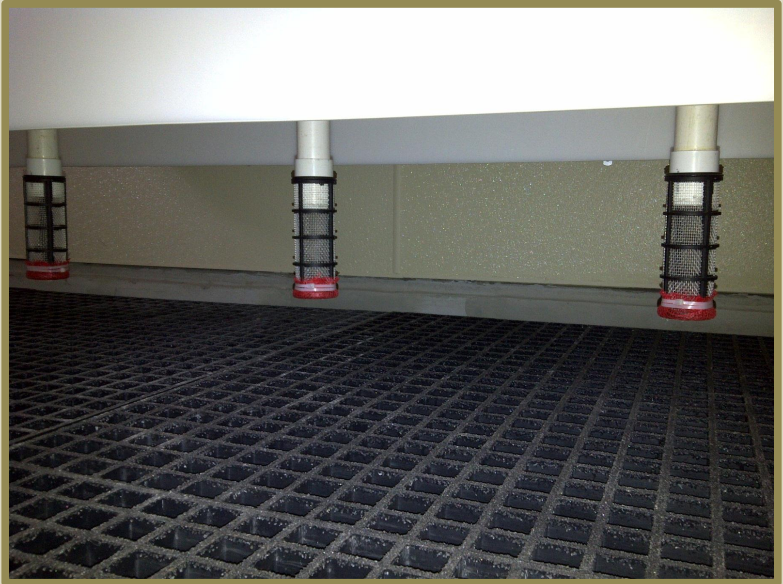
Filters- Attached to each drain are modified pump filters to catch debris washed out during the delinting process to prevent pump malfunction.
