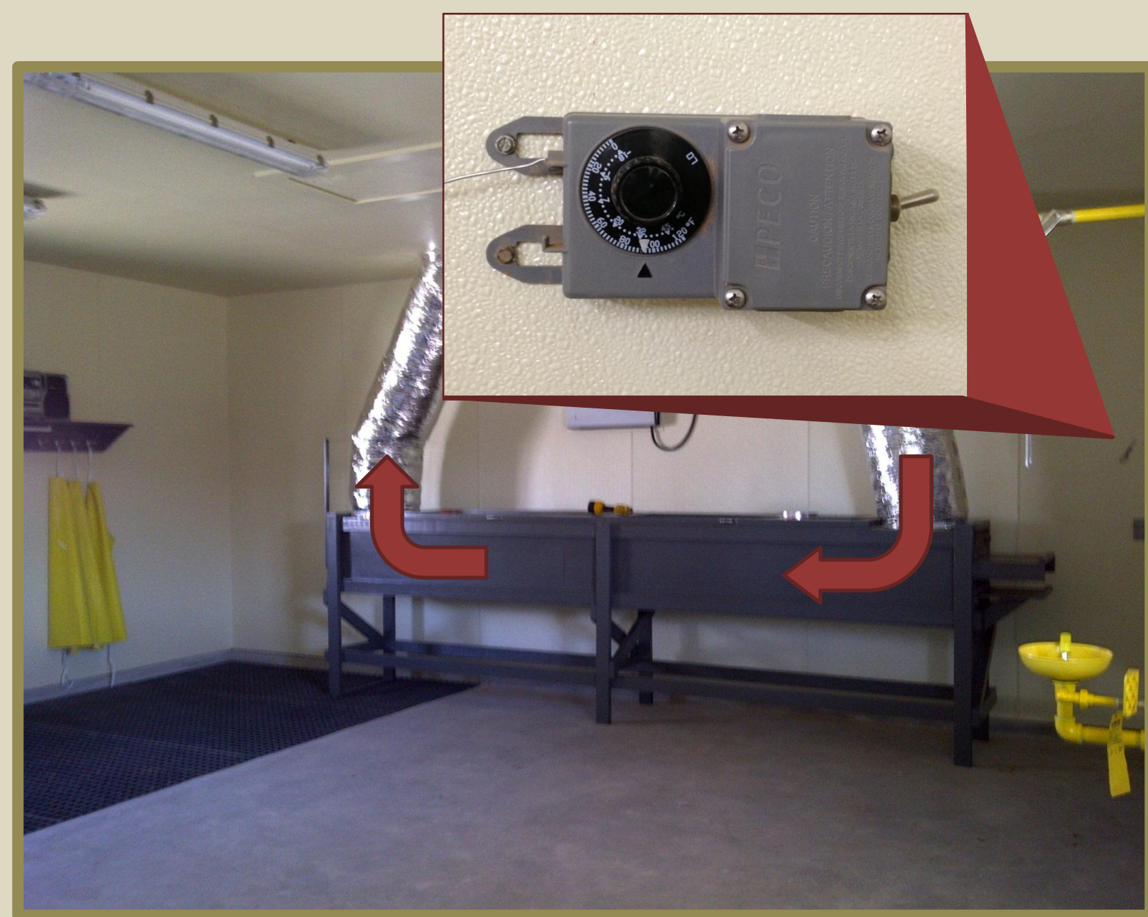
Thermostat- A sensor directly placed in the box allows the thermostat to keep the temperature at any desired setting. A switch to manually turn on the fan was installed if no heat was desired to dry the seed. With the return air pulling the warm air directly from the dryer box the heating unit itself is not required to run continuously making the dryer more efficient.
