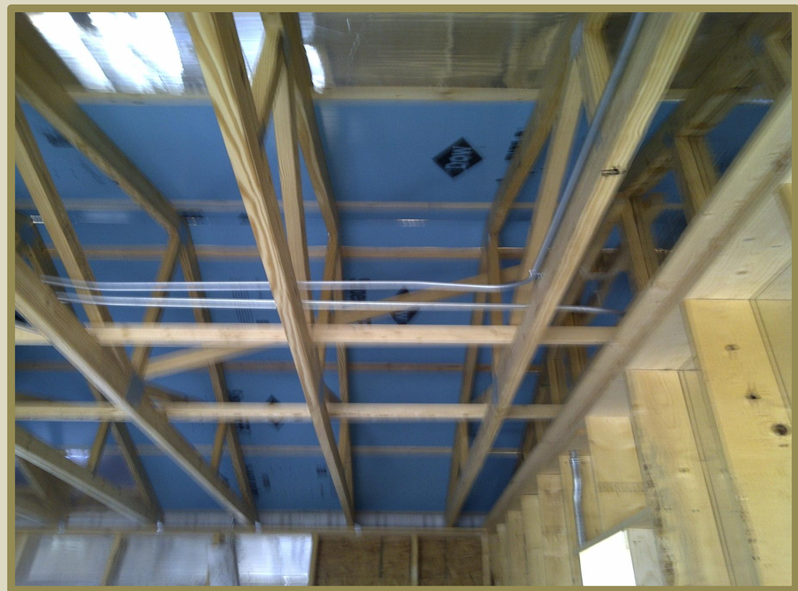
Rafters- Built to specific dimension, the rafter allows for the heating unit to be tucked away in the attic space.
