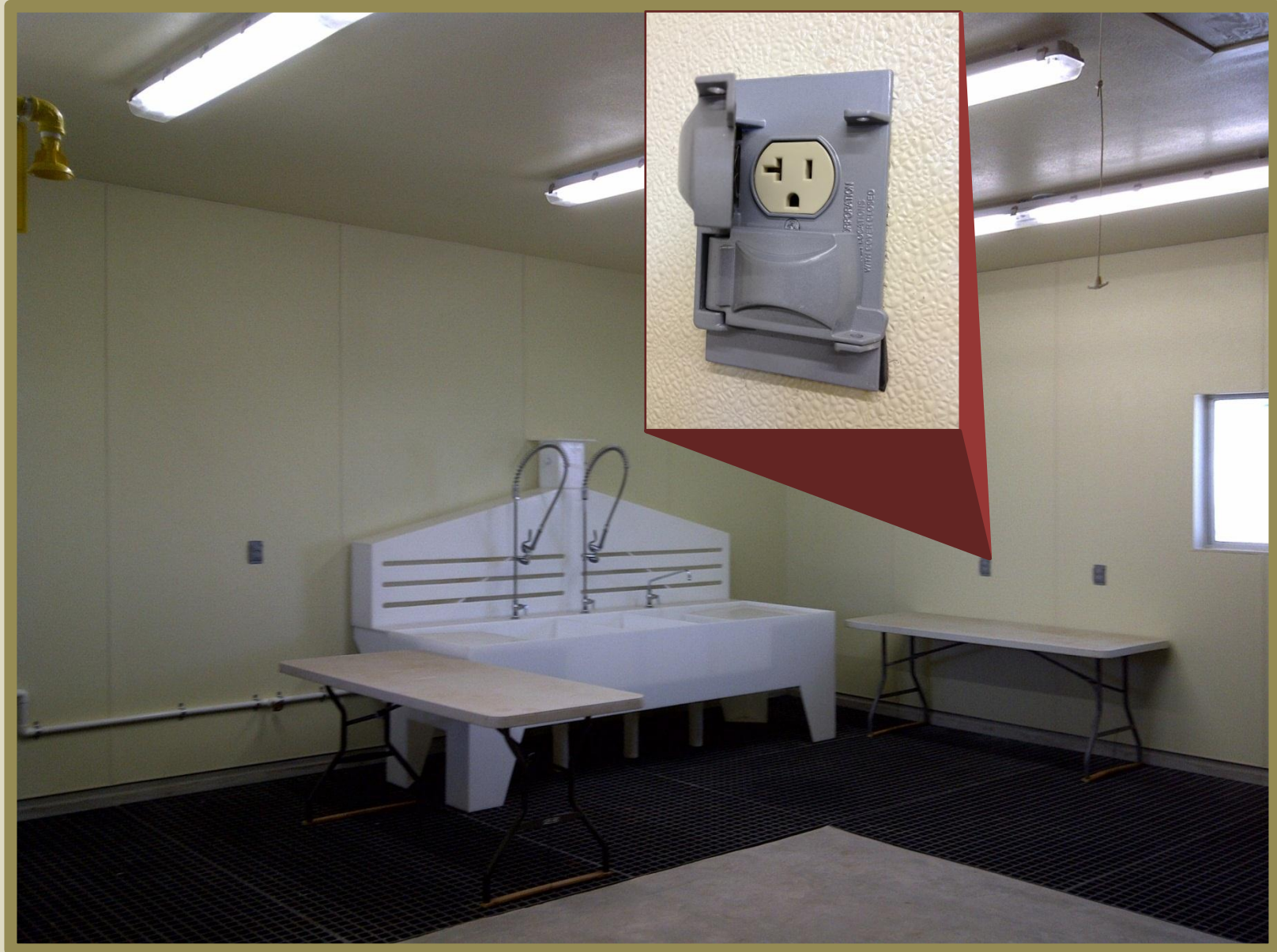
Sink- The sink is made of a poly material resistant to corrosion with 3 separate wash areas for different stages of the delinting process. Electrical Outlets- The outlets are all covered for water resistance to allow interior walls to be sprayed down without damaging or tripping the electrical system.
