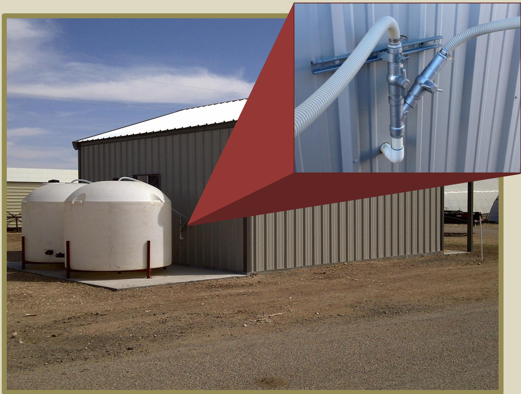
Tanks- Two 15,000 gal tanks are split with a y-valve to allow the waste water to be diverted to either tank.
