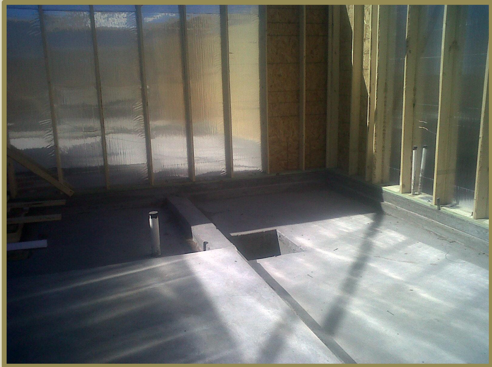
Sloped Foundation- The reinforced concrete foundation was poured at a specific slope to ensure proper drainage of acid water and debris. The sloped area was split into 2 parts to allow adequate support for the grated flooring. A 2inch by 1inch lip was given on the inner perimeter of the sloped area to allow the fiberglass reinforced poly grated flooring to be installed.
